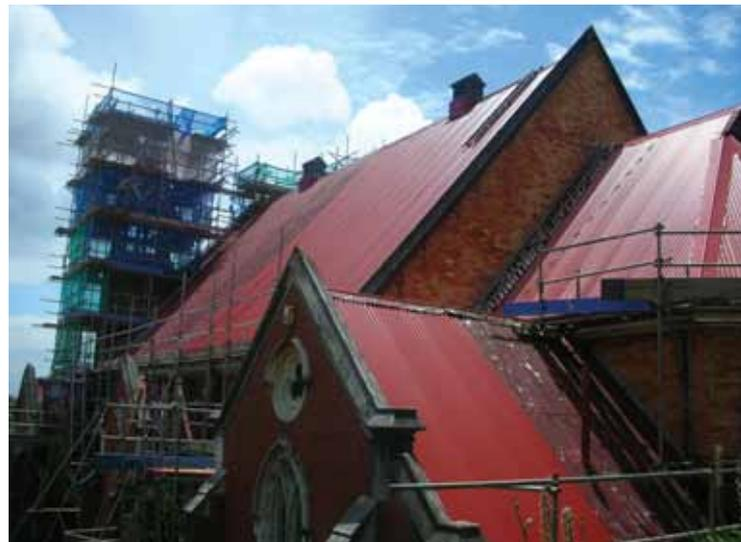
demanding physically with every single sheet having to be loaded into position by hand due because no machinery could be deployed. Metro roofers Callum Page, Ken McDonald and James Rutten, using rope harnesses, managed to install six sheets per day on the 55 degree pitch roof.
